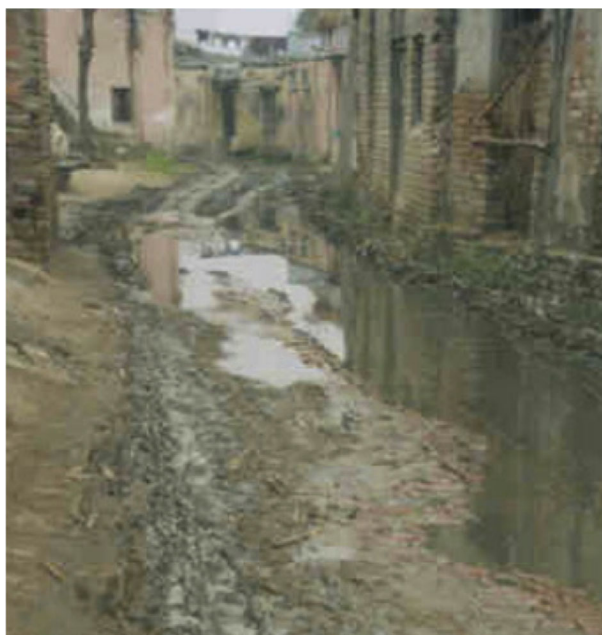
FIGURE A1 An overflowing drain in one of the sampled villages (Haridwar, Uttarkhand) [Colour figure can be viewed at wileyonlinelibrary.com ]
